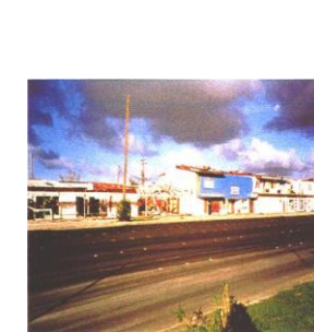
Weakened wood and tin roofs can fail
