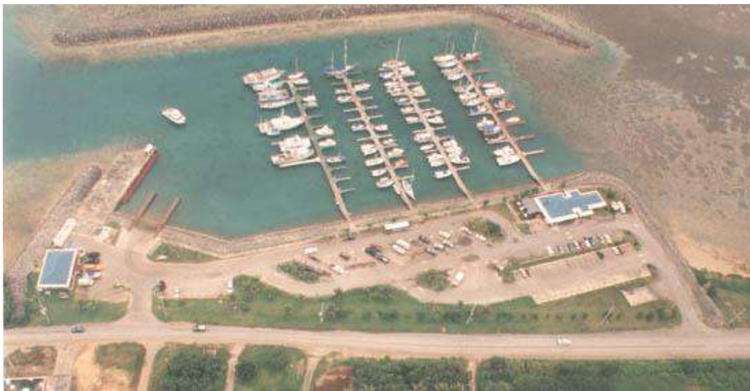
Figure 2. View of Agat Marina from the air showing the marina entrance at the left, the four docks and the 99 slips. The building at the right (blue roof) is the restaurant and the building at the left (blue roof) is the marina operations office. (Picture taken from www.portofguam.com )
