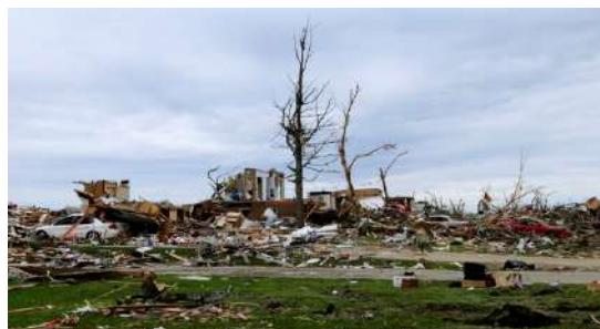
Figure 11. Debris on Private Property
